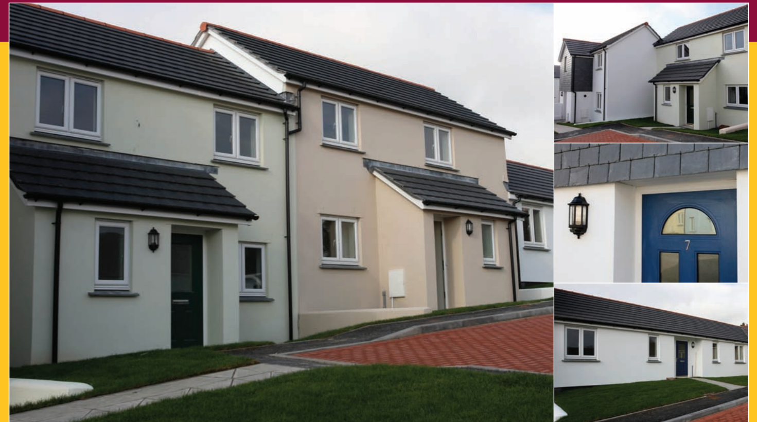
Just a few of the new homes completed at Pentowan Gardens - Hayle.
